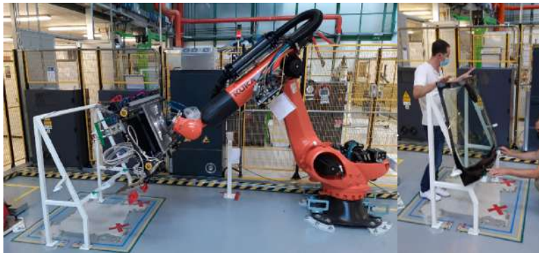
Figure 10: CRF Robot workcell installation.
